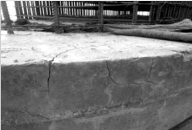
Fig. 3 Plastic Shrinkage Cracks of Deep Depth
