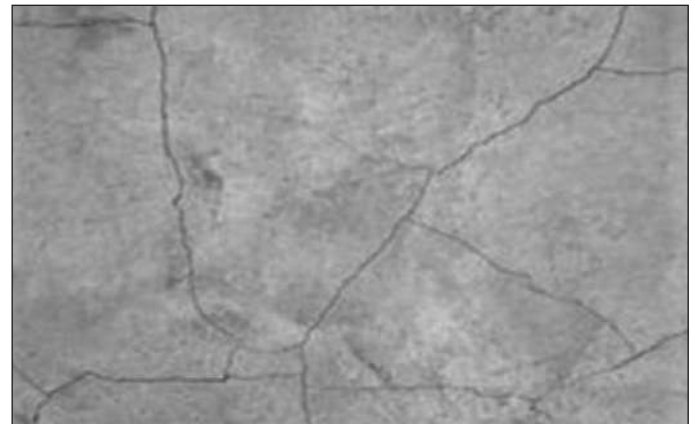
Fig. 2 Plastic Shrinkage Cracks of Shallow Depth
